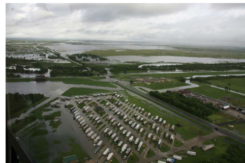
Aerial photo of the Hillebrandt area of Jefferson County immediately after Hurricane Harvey, Beaumont Enterprise
